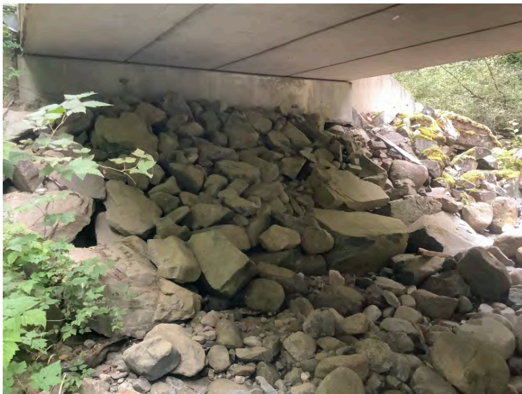
Right Bank Abutment when facing downstream
