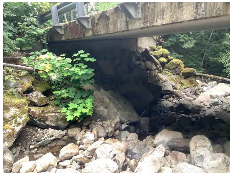
Left Bank Abutment when facing downstream
